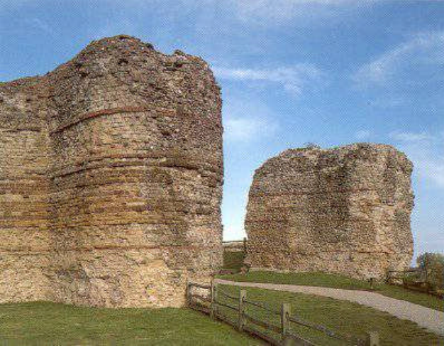
Pevensey: massive Roman towers on the West Gate
