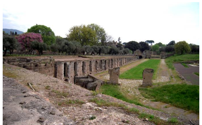
Service Quarters, or Cento Camerelle , from the north. On centre right is the paved ring road, unearthed in 2000. Photo F Radcliffe 2009 ©
