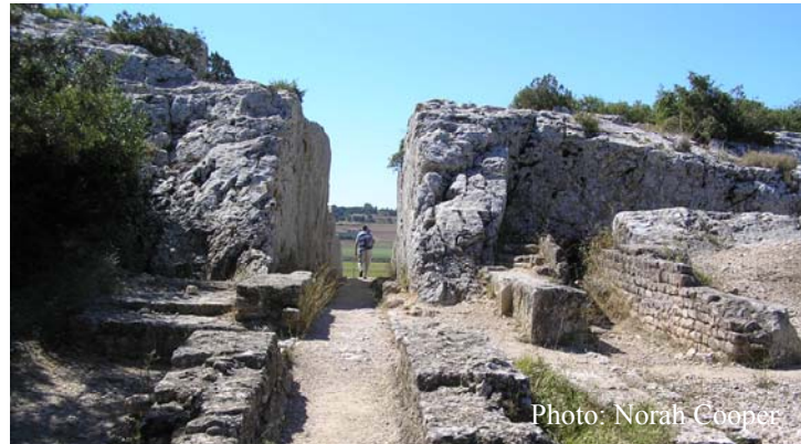
Cut through rocks for second aqueduct to top of Barbégal. Wall on right shows 90° turn of first aqueduct to Arelate
