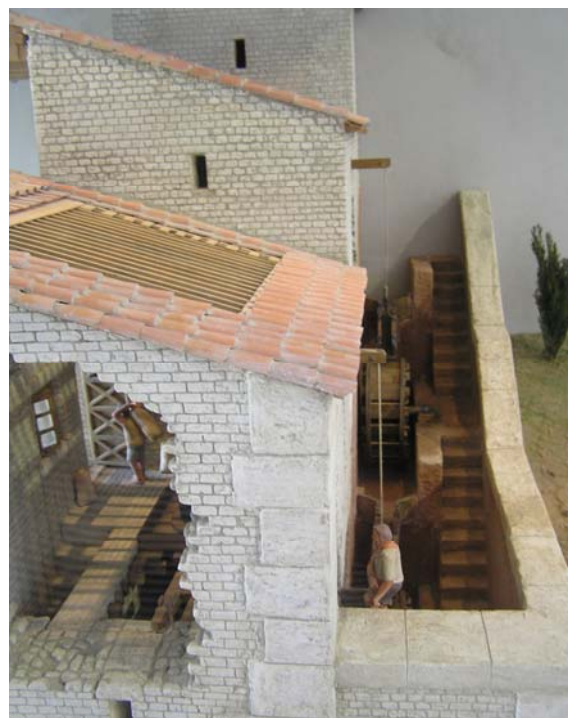
Model of part of mill showing overshot waterwheel: Arles Museum
