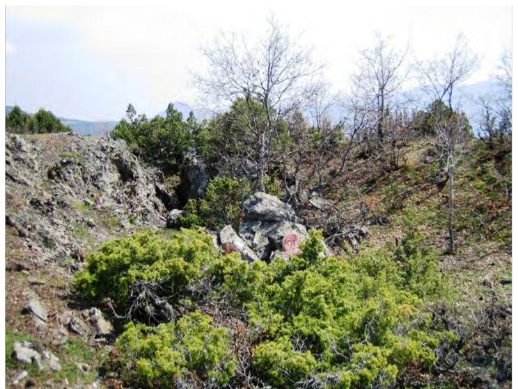
Figure 1. Collapsed old workings at Derinin Tepe
