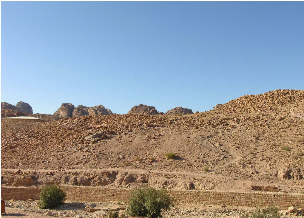
Figure 3. The southern slope of the NEPP area, featuring the facade-like structures (Photograph by Zbigniew T. Fiema).
