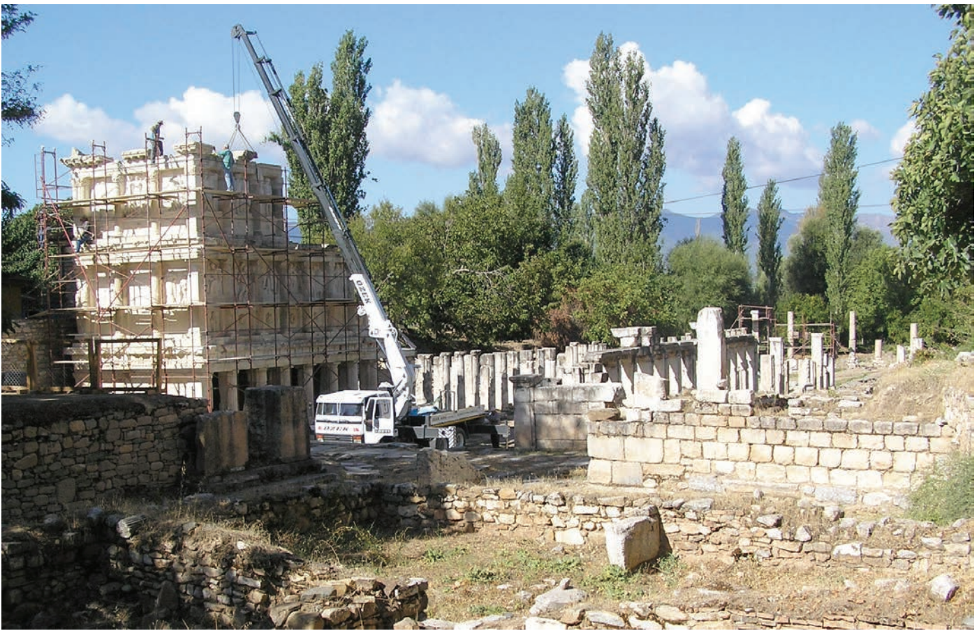
The Sebasteion under restoration.
