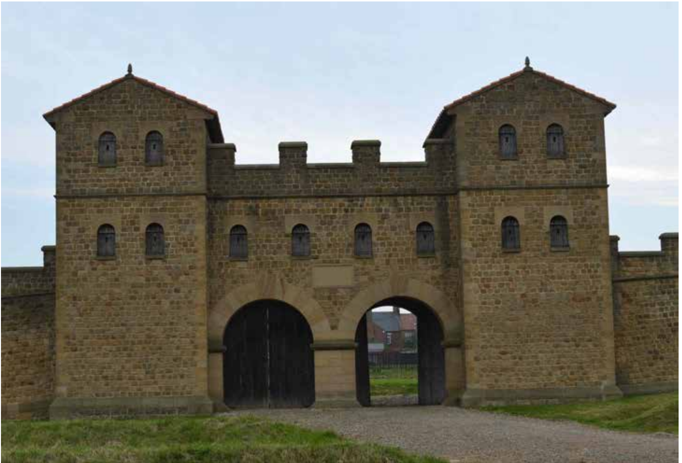
West Gate (reconstructed) of the fort at South Shields, supply base for the Severan campaign in Britain.
