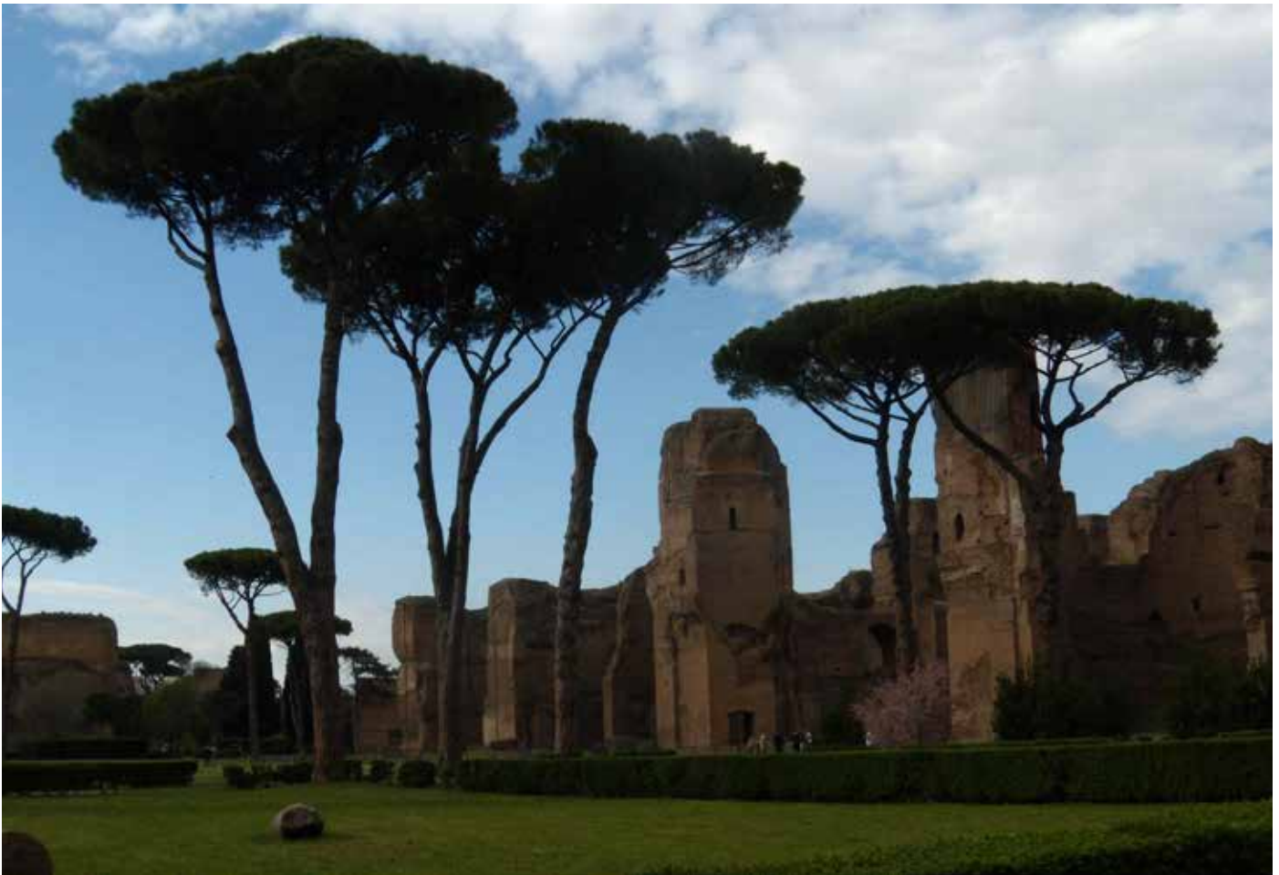
The Baths of Caracalla in Rome. AD 211-16. Now a vast ruin with almost all its marble veneers removed. The walls and vaults required 210,000 cubic metres of concrete and millions of bricks. There were 252 columns, sixteen of which weighed over 50 tons each. Photograph: Guy de la Bédoyère.
