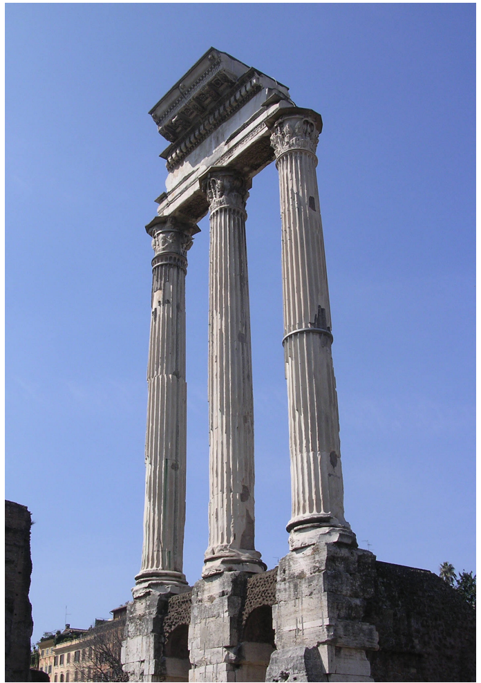
A close-up view of the columns. Note the weight-relieving alcoves between the columns' substructures in the podium. Perhaps the raven lived in one of these.
